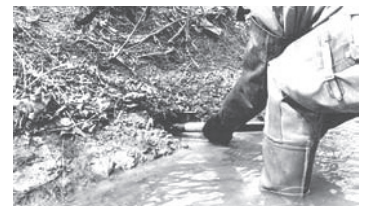
Dig pocket at water line
